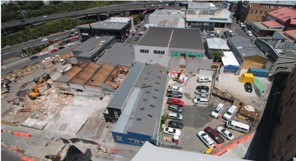
To minimise dust a portable water mister and water hoses are being used. Noise, vibration and air quality monitors are also in place to ensure we stay within our consented limits.
